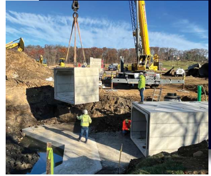
The Glens of Jackson Township Setting Box Culvert with Crane Jackson Township
