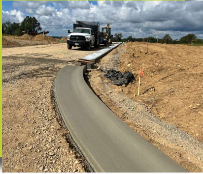
Oldstone Crossing No. 3 Placing New Wet Concrete Curbs Lake Township
